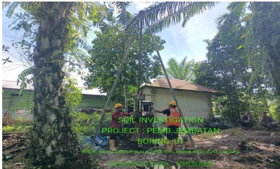
Pemasangan Standart Penetration Test (SPT)
