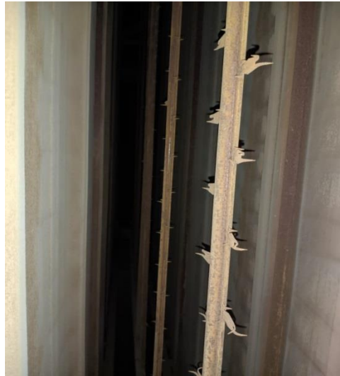
Gambar 2. 7 Discharge Electrode (DE)
