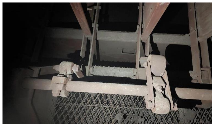
Gambar 2. 10 Rapper/Rapping System
