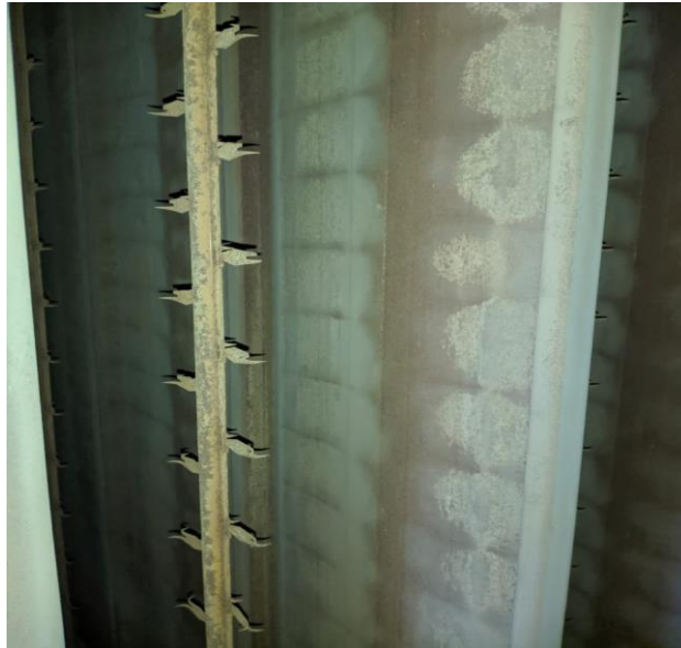
Gambar 2. 6 Collecting Electrode (CE)
