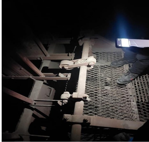
Gambar 2. 8 Hammering Device (HD)
