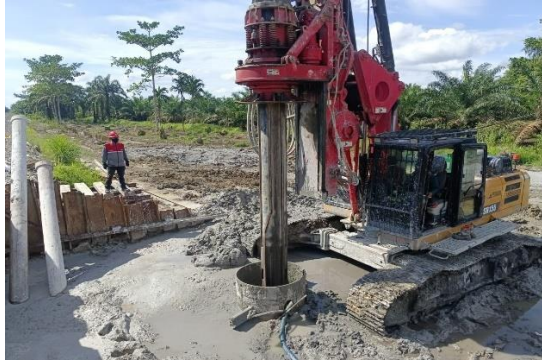
Gambar 2. 2 Bored Pile
