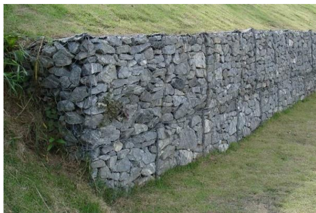
Gambar 2.11 Tembok Penahan Tanah Gabion
