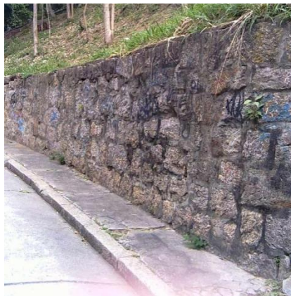
Gambar 2.5 Tembok Penahan Tanah Gravity
