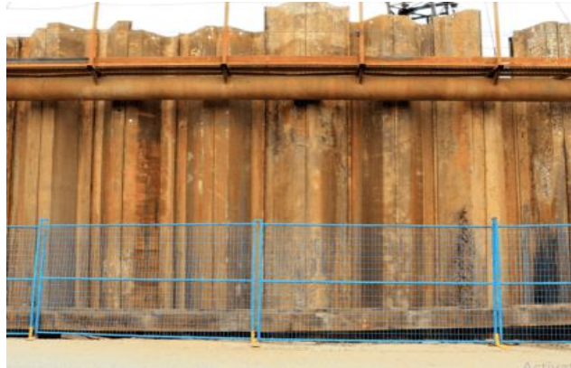
Gambar 2.8 Tembok Penahan Tanah Sheet Pile
