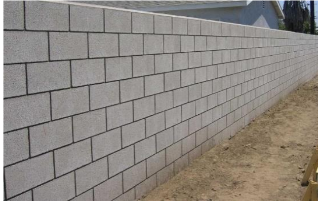
Gambar 2.10 Tembok Penahan Tanah Beton
