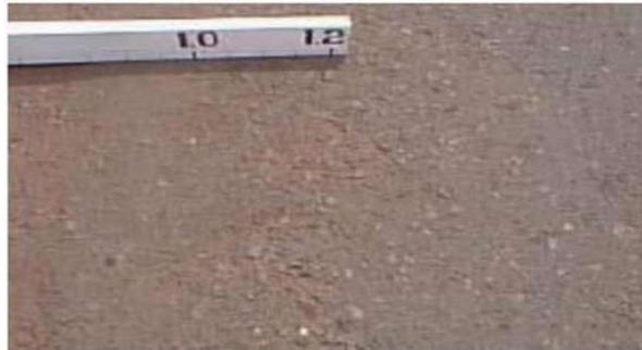
Gambar 2.12 Pengausan Agregat ( Polished Agregat ) Sumber : Bina marga no.03/MN/B/1983
