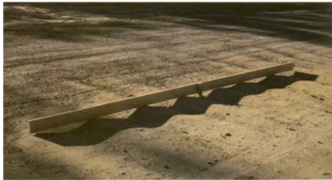
Gambar 2.5 Keriting ( Corrugation ) Sumber : Bina marga No.03/MN/B/1983
