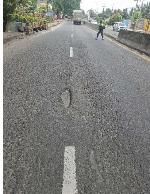
Lubang ( potholes )
