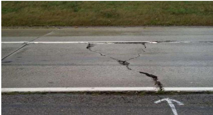
Gambar 2.5 Retak Sambung Bahu Perkerasan (Shahin, 2005)
