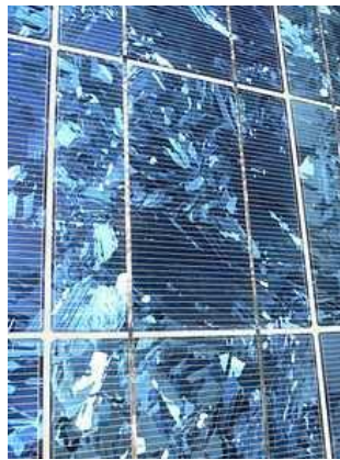
Gambar 2.10 Panel Surya Polycrystalline Silicon
