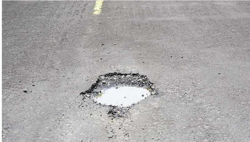
Gambar 2.11 : Lubang (Pothole)
