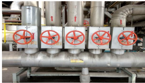
Gambar 2.18. Steam header
