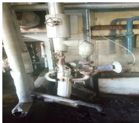
Gambar 2.23 Auto & manual blowdown valve
