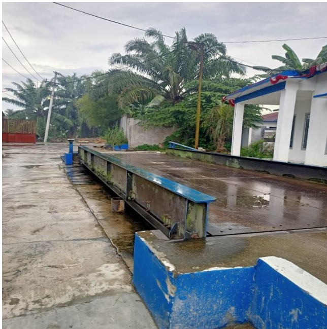
(a) Weighbridge (jembatan timbangan)
