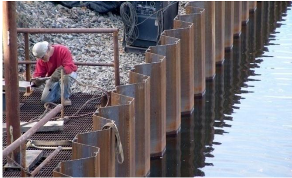
Gambar 2.12 Dinding penahan tipe Sheet pile (Sumber : regainindustrial.com )
