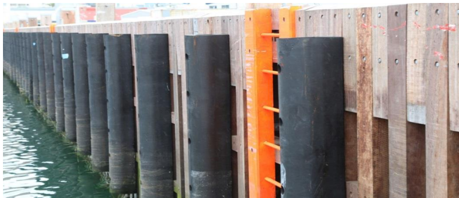
Gambar 2.20 Fender tipe D (Sumber : Shibata Fender Team)
