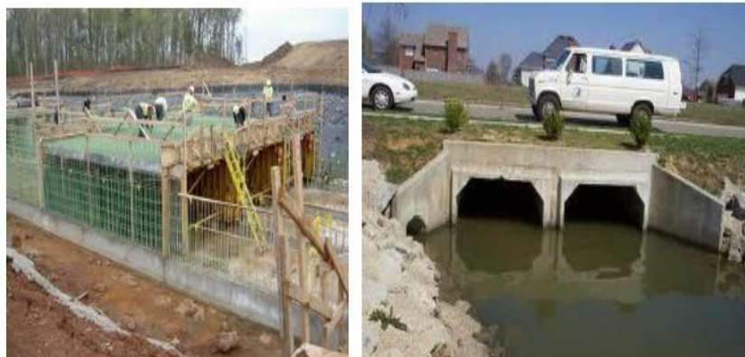
Gambar 2.15. Box Culvert cast in place
