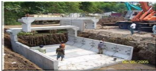
Gambar 2.19. Reinforced Concrete Box Culvert Box (RCBC)
