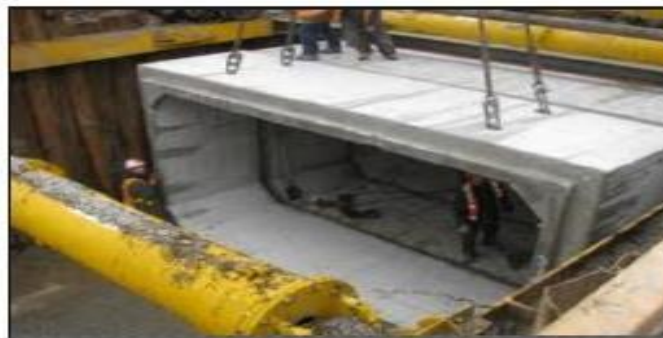
Gambar 2.14. Box Culvert Precast
