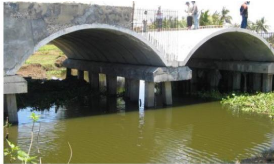
Gambar 2.16. Arch Culvert
